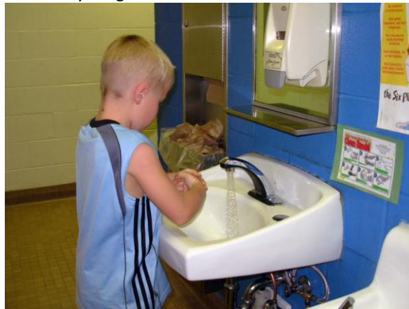
Ethan H. tries out the new touchless water faucets in the south hallway sinks. The touchless faucets were installed in both the north and south hallway bathrooms.
